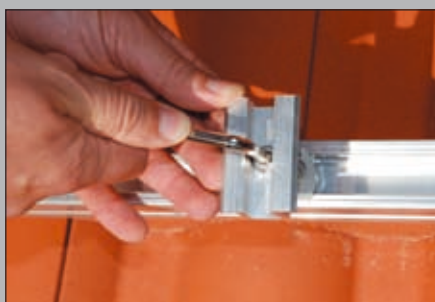
5 - Insert the PMF and PMC clamps
