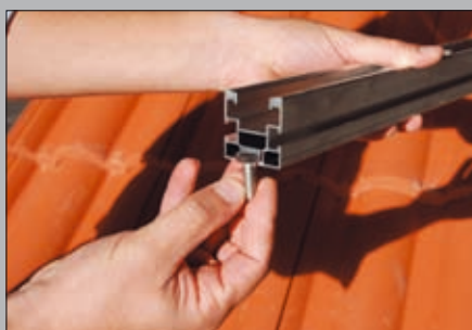
2 - Insert the screws into the Solar-Plus profile
