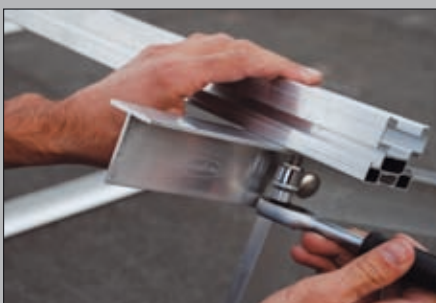
4 - Clamp the Solar-Plus profile to the frame
