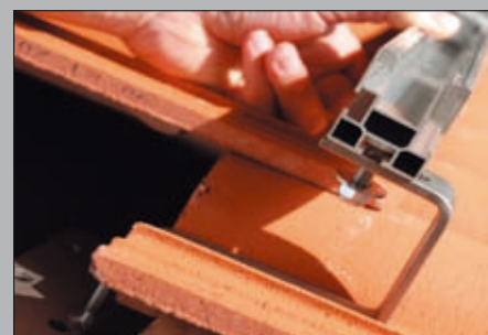
3 - Place the Solar-Plus into the hook
