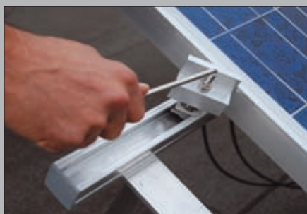
5 - Insert the PMF and PMC clamp
