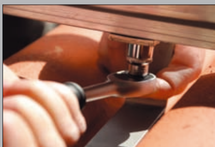
4 - Clamp the Solar-Plus profile to the hook
