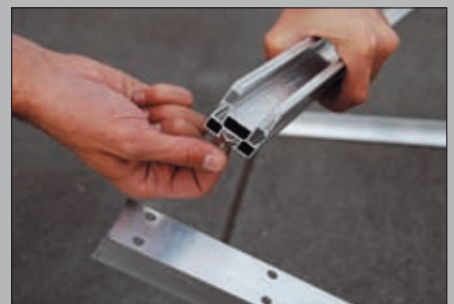
3 - Insert the screws into the Solar-plus profile
